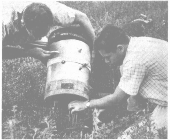
Clipped stems within nozzle shaken to loosen insects.
