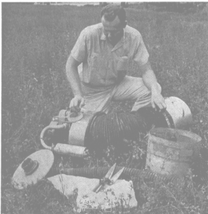
Portable machine for sampling field insect populations.
